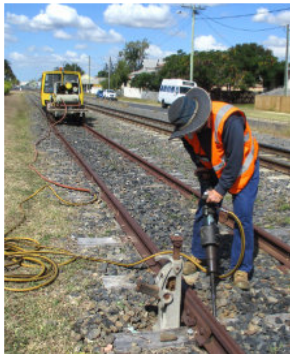
John Kennedy working with the tamper, 23 May 2021.
