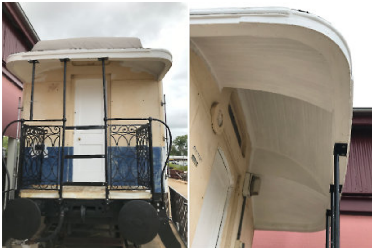
Recent exterior repair work on CWM21.
