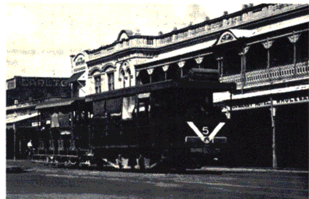
Coming (on the left) and going (on the right) as indicated by the large V and inverted V respectively on the car ends. This innovation was in use for some time in the 1930's.
