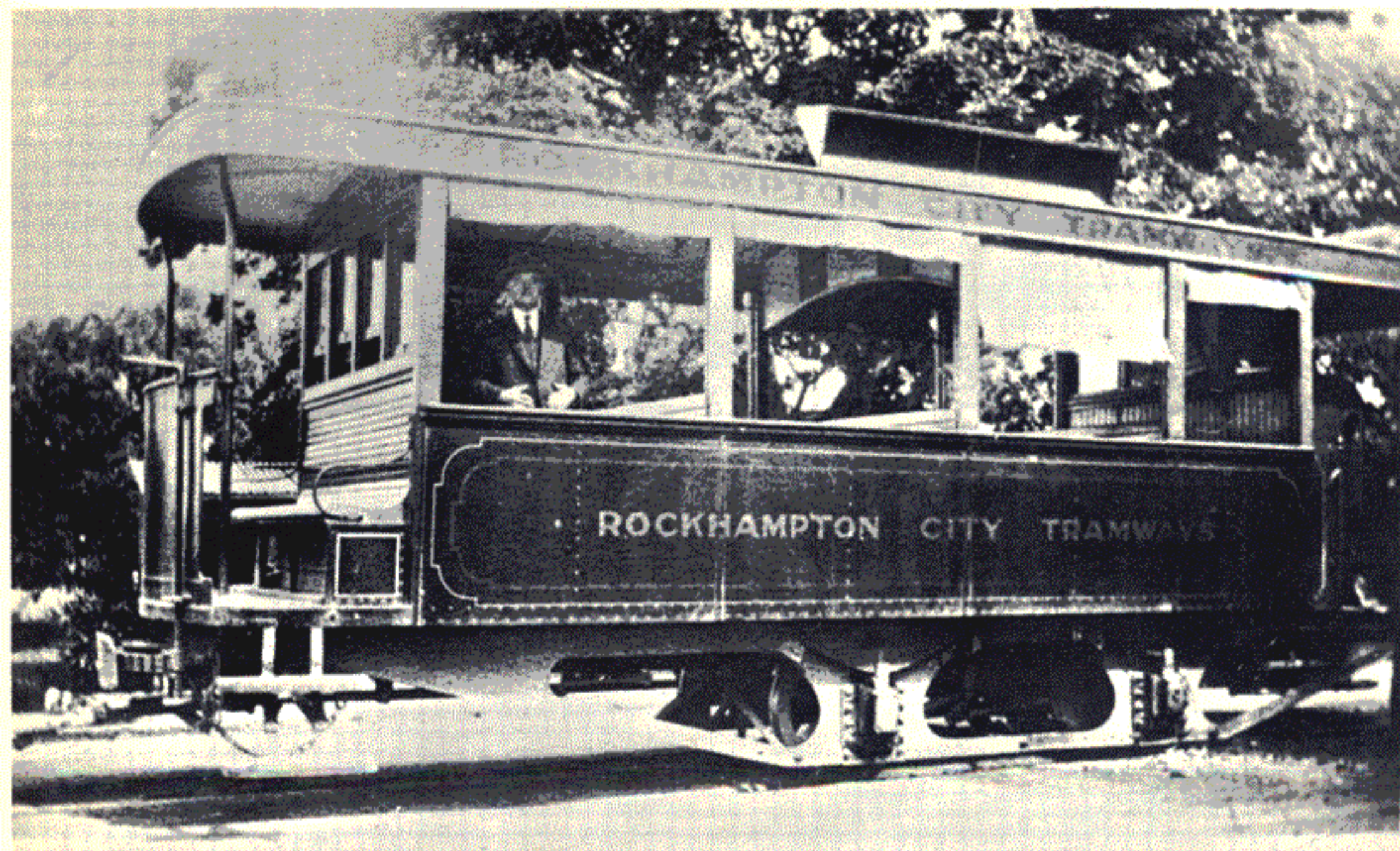
This view of car No. 7 at Gardens in 1929, shows clearly the interior transverse roof strengthening arches and the reflected light roof mounted advertisement. (Photo: B. Dion)
