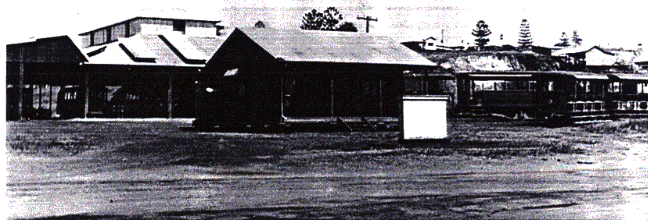
A depressing scene three months after closure as both motors and trailers lie disused inside and outside the depot awaiting their final disposal. (Photo: D. Murray)
