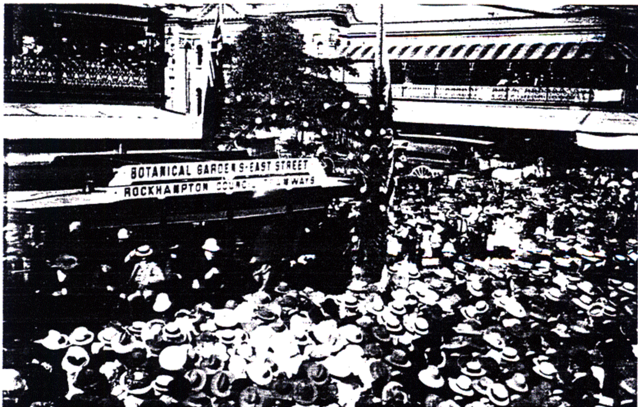
The leading car of the two available on the opening day passes through the ceremonial arch and breaks the opening ribbon on 5th June, 1909. (Photo: J.W. Knowles' Collection)
