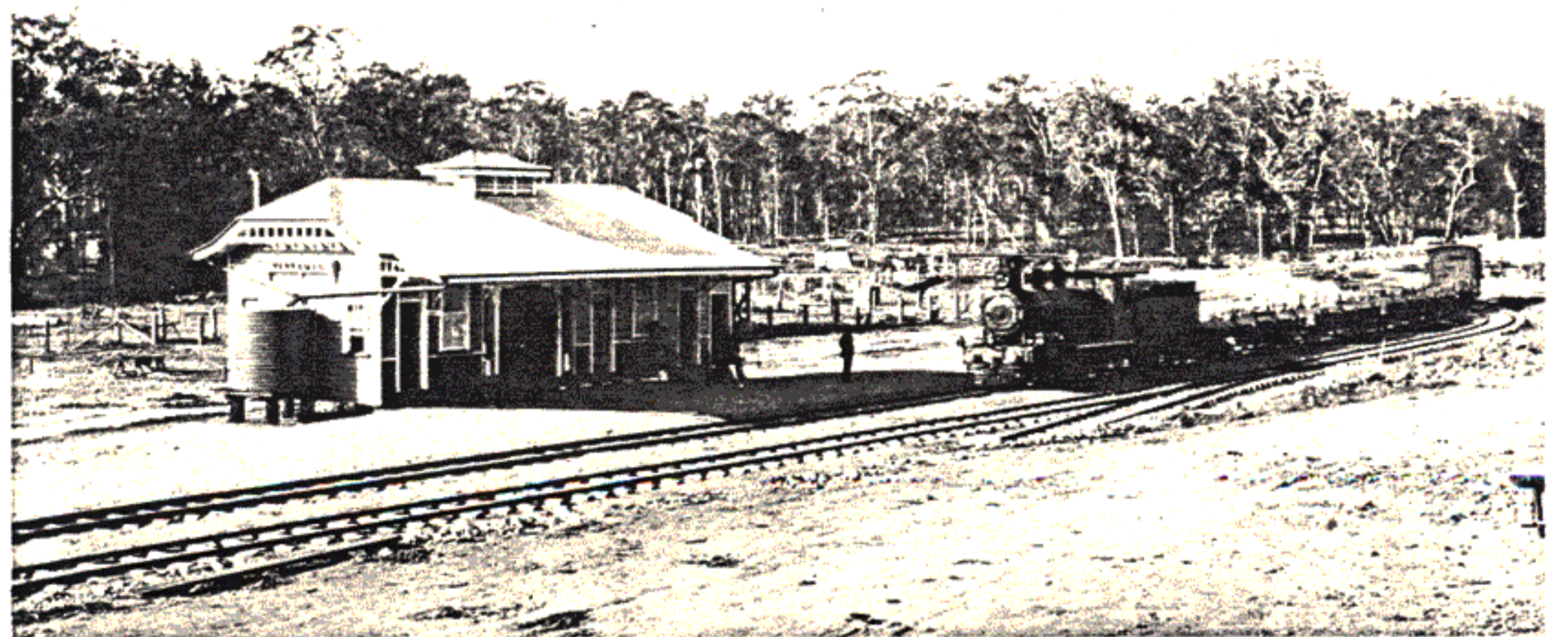
Yarraman, a typical Queensland Railways' branch-line terminus, in 1913, with a B.15 Converted 4-6-0 on a construction train. (Photo: Queensland Railways)
