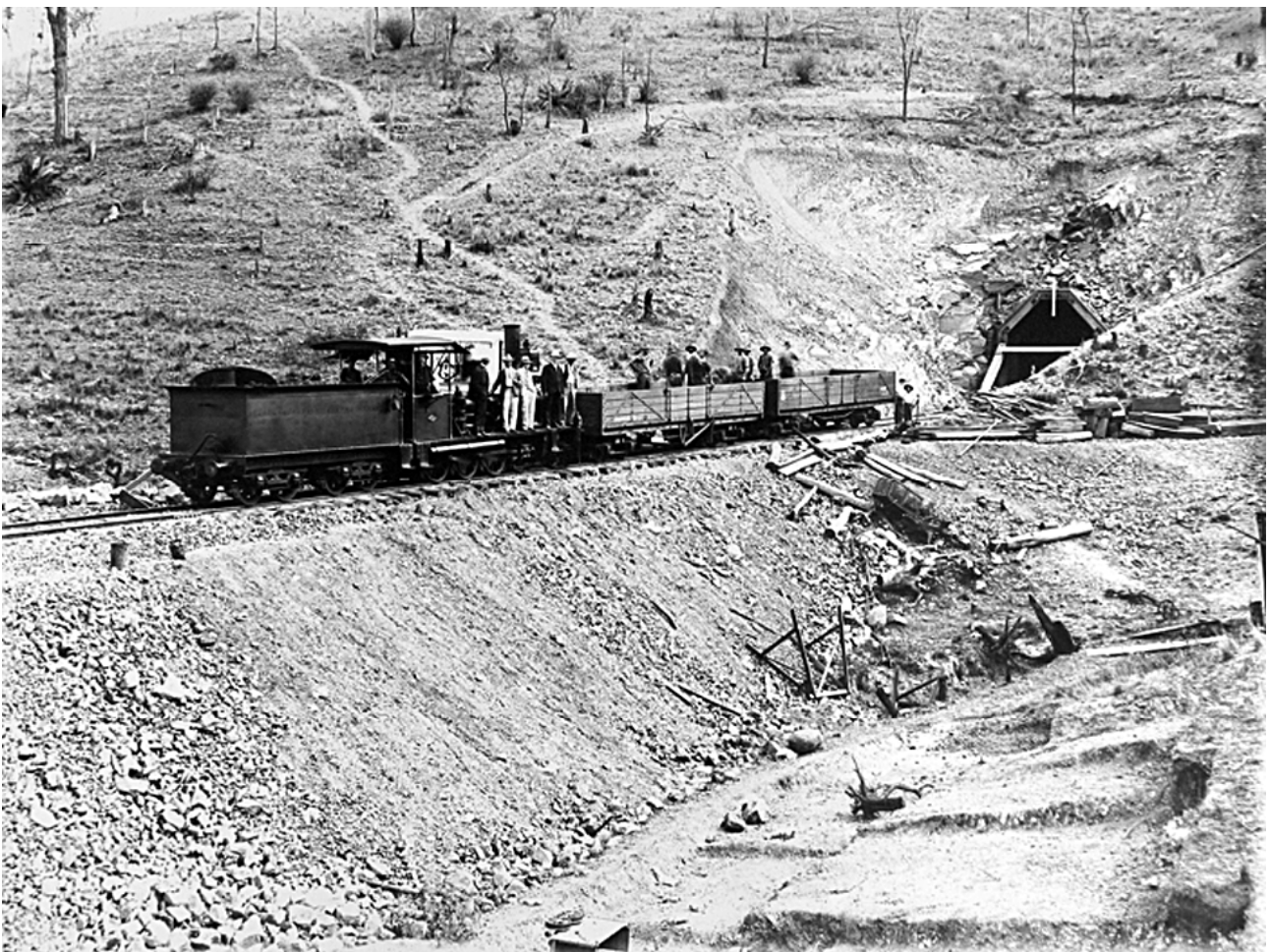
Contractor's locomotive and 3' 6" gauge 'H' wagons during construction of the Linda Gully Bridge tunnel for the No 2 Branch. Mount Morgan Rail Museum ppt Collection, Jens Hansen Lundager photographer.
